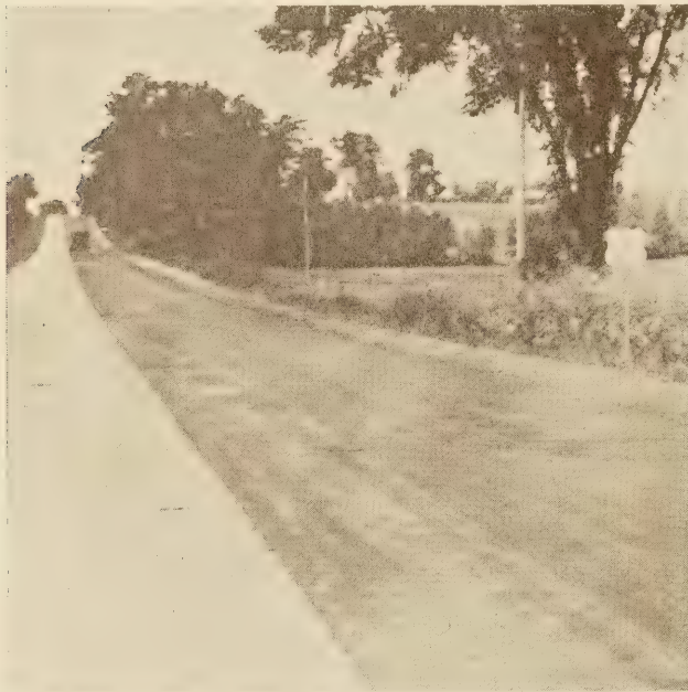
FIGURE 5.—SECTION IN GOOD CONDITION THREE MONTHS AFTER TREATMENT. THE SURFACE CONTAINED AN APPRECIABLE AMOUNT OF MOISTURE WHEN OIL WAS APPLIED
